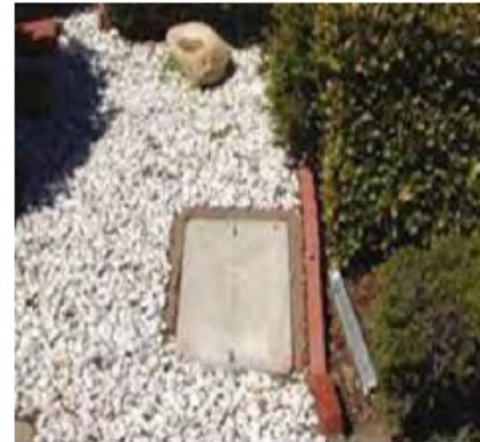
TYPICAL SPECTRUM/CROWN CASTLE HANDHOLE
