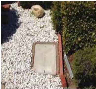
TYPICAL SPECTRUM/CROWN CASTLE HANDHOLE
