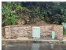
NEW Retaining Wall by City
