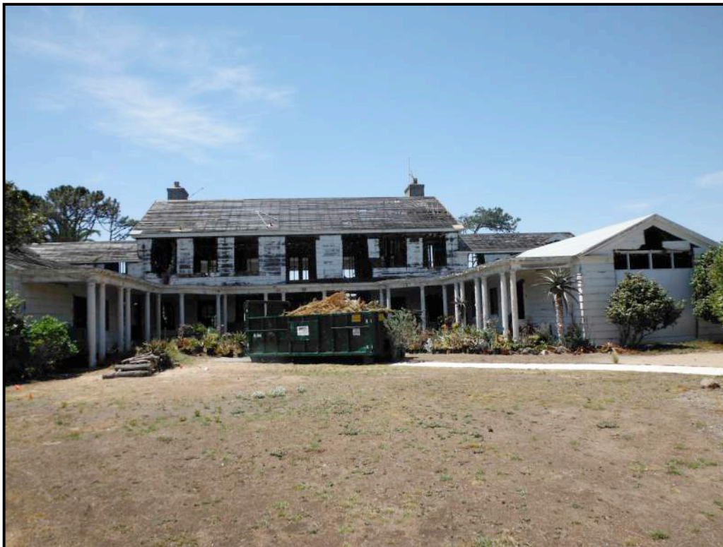
Plate 4.1-2: Tippet Hall circa 2014 after being gutted and partially demolished.
