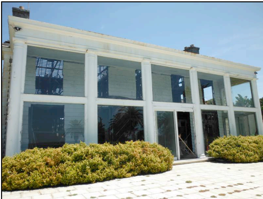
Plate 4.1-4: Glass windows installed to enclose the rear porch.
