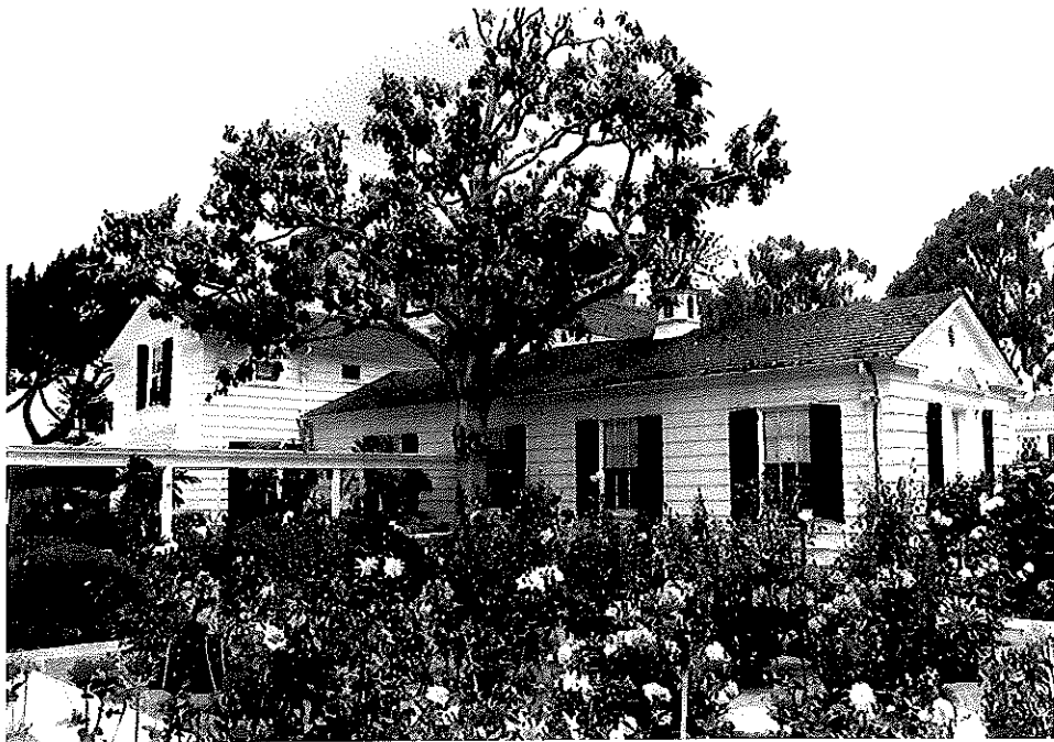
Photograph #14 Tippett Hall Southeastern Garden View Facing Northwest
