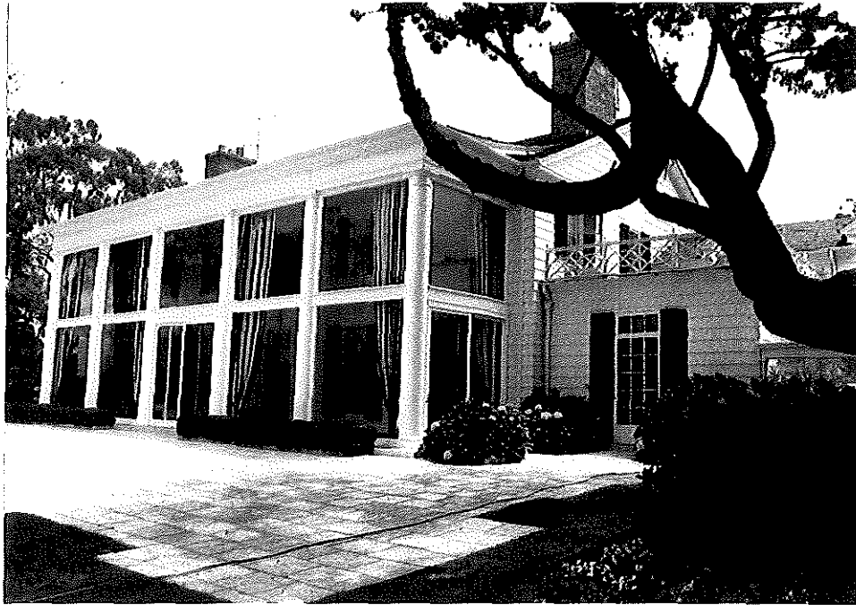
Photograph #11 Tippett Hall Western Elevation View Facing Northeast
