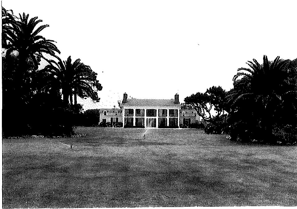
Photograph #9 Tippett Hall Western Elevation & Grounds View Facing East
