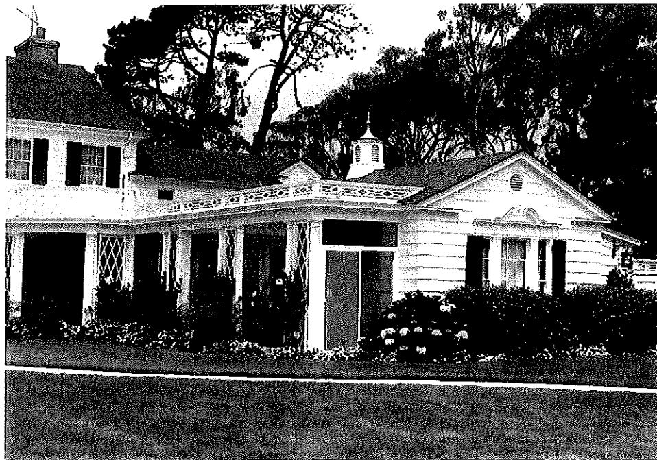
Photograph #4 Tippett Hall Eastern Elevation Northern Ell View Facing West
