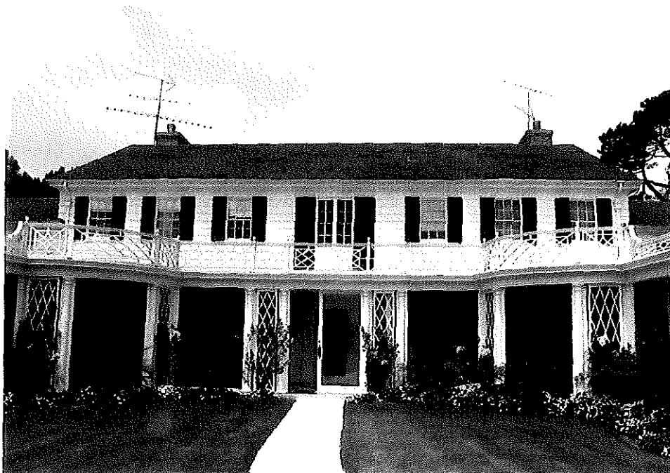
Photograph #2 Tippett Hall Eastern Elevation View Facing West
