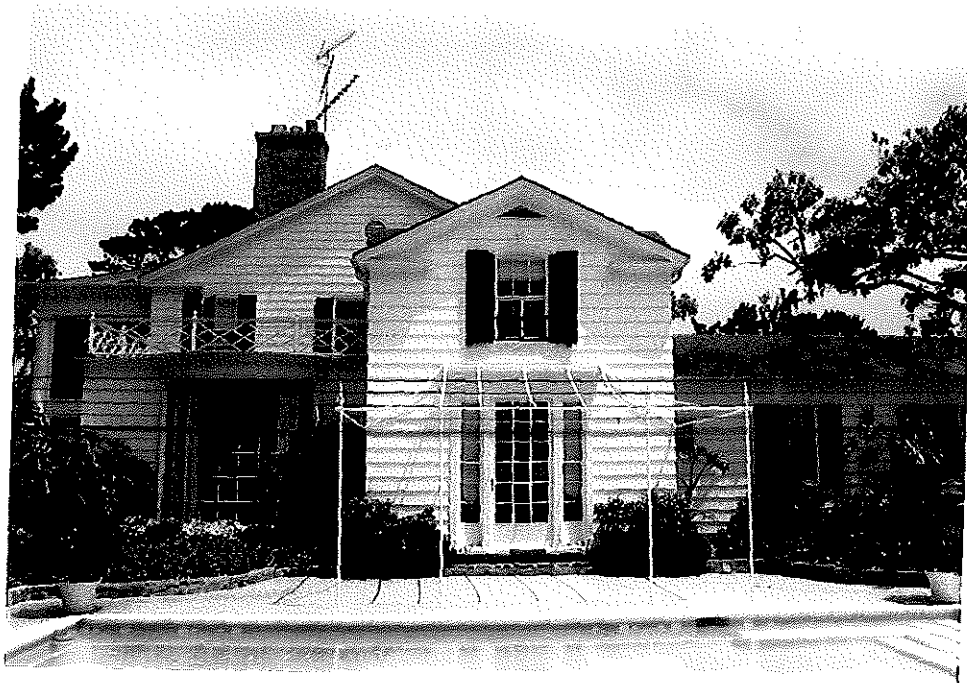
Photograph #8 Tippett Hall Southern Elevation View Facing North
