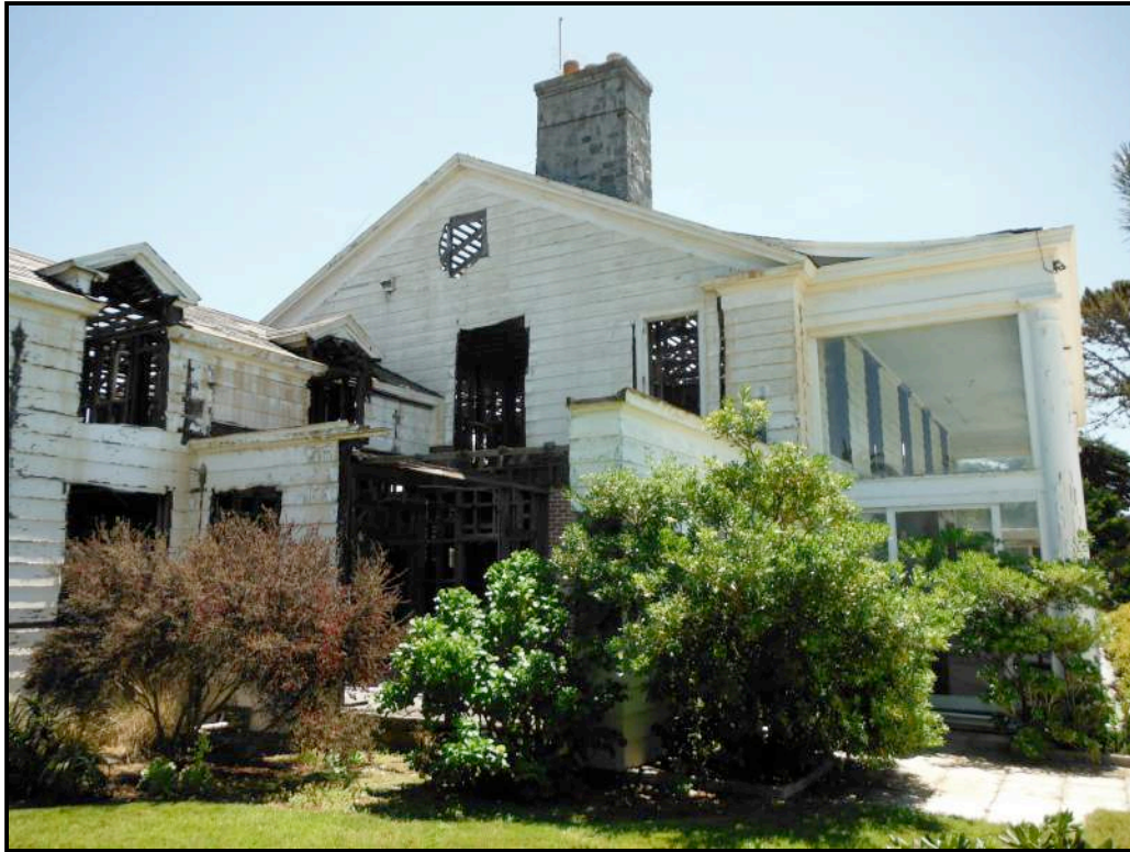
Plate 4.1-3: View of the low-pitched, side-gabled style of the roof. Note the cornice lines emphasized with a wide band of trim. The effects of demolition since 2000 are obvious.
