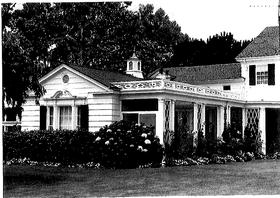
Photograph #3 Tippett Hall Eastern Elevation Southern Ell View Facing West
