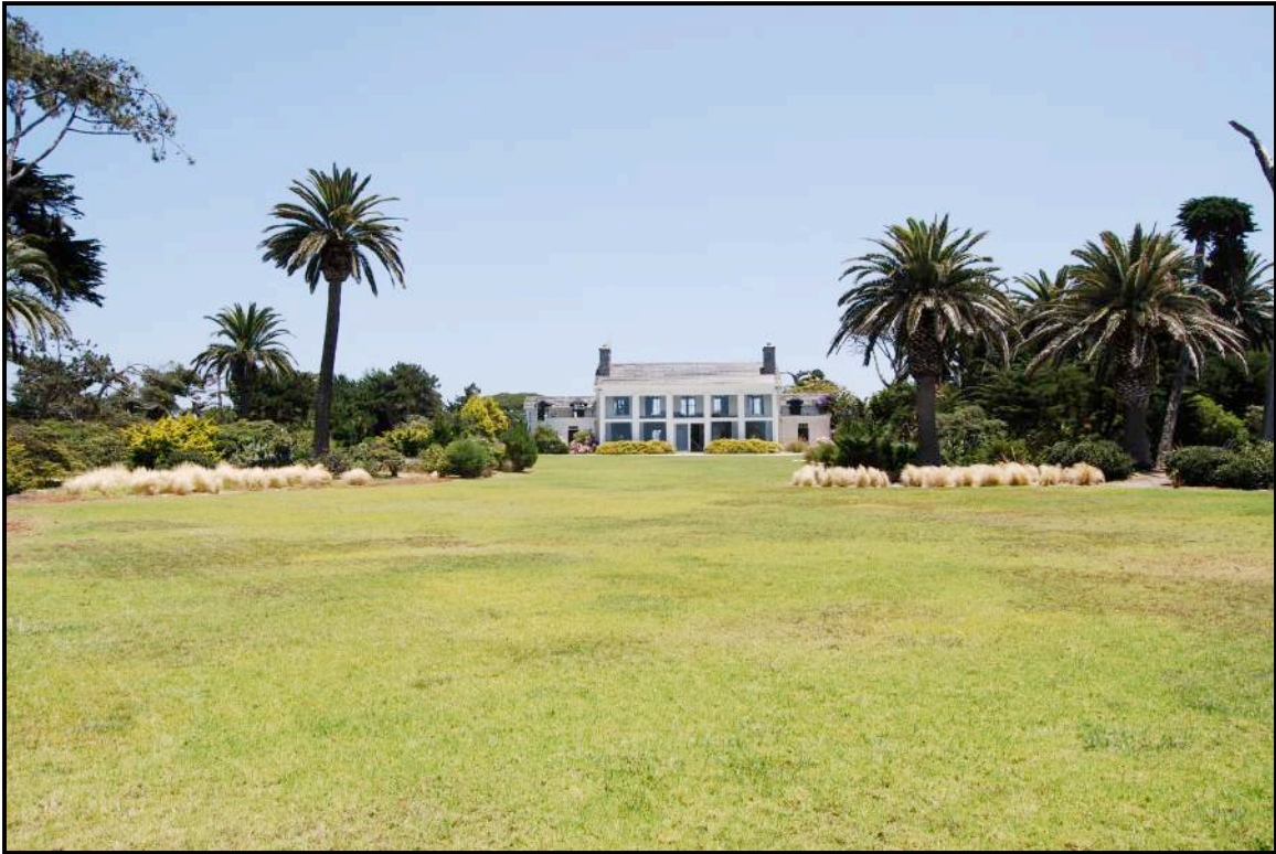
Plate 3.1–3: View of the backside of Tippett Hall, facing east.
