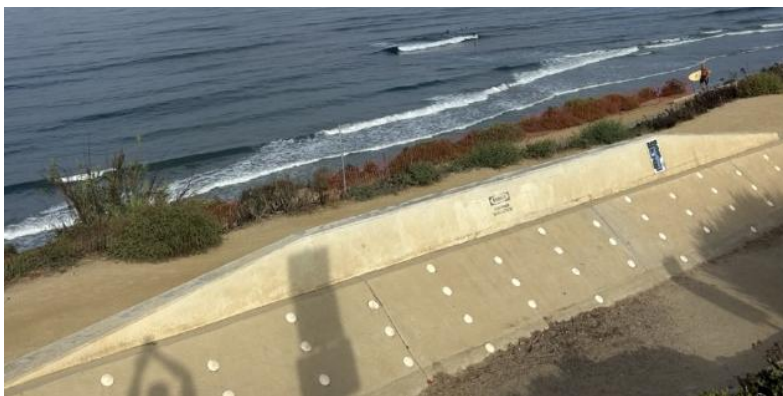
A splash wall behind the drainage channel near 7th Street.
