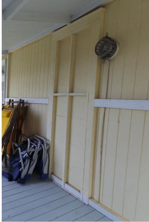
119 10 th Street, Del Mar September 2017 Photograph #21 View of enclosed window on the west façade
