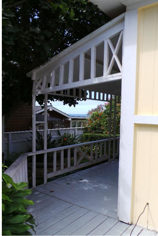
119 10 th Street, Del Mar September 2017 Photograph #23 View of porch detailing
