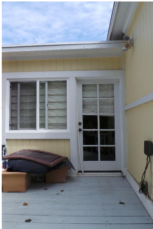
119 10 th Street, Del Mar September 2017
