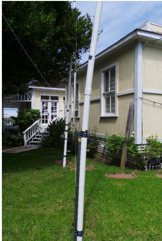
119 10 th Street, Del Mar September 2017 Photograph #38 View north of rear of main cottage and corner of rear addition
