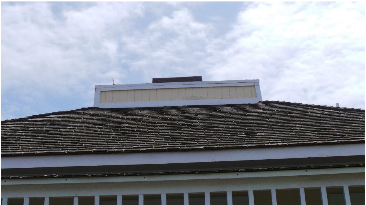
119 10 th Street, Del Mar September 2017 Photograph #6 View of south of faux widow's walk
