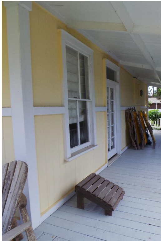
119 10 th Street, Del Mar September 2017 Photograph #18 View south along the west façade
