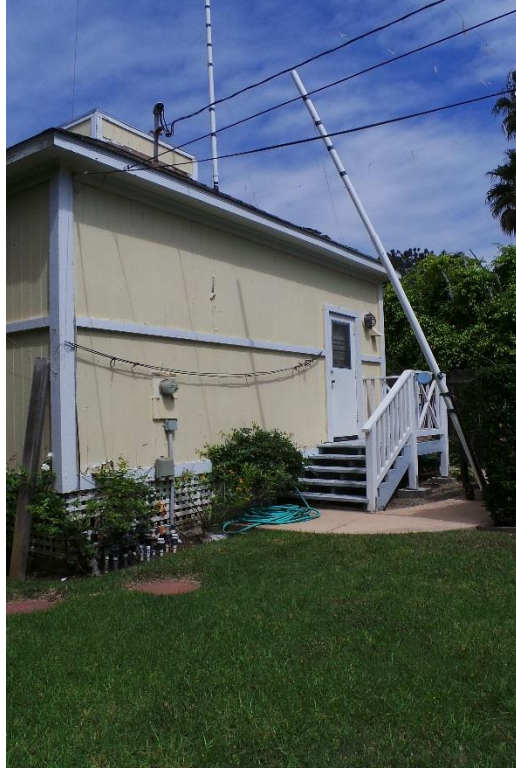
119 10 th Street, Del Mar September 2017 Photograph #39 View northeast of rear addition
