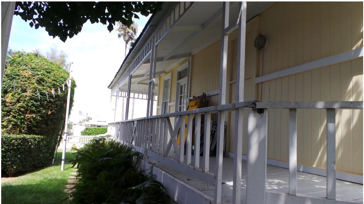
119 10 th Street, Del Mar September 2017 Photograph #24 View north of porch along the west façade
