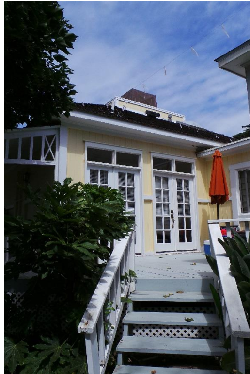
119 10 th Street, Del Mar September 2017 Photograph #26 View northeast of stairs to access balcony
