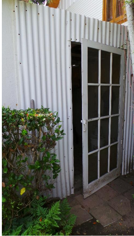
119 10 th Street, Del Mar September 2017 Photograph #51 View of entrance to garage
