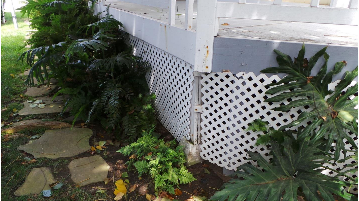
119 10 th Street, Del Mar September 2017 Photograph #25 View of trellis covering foundation
