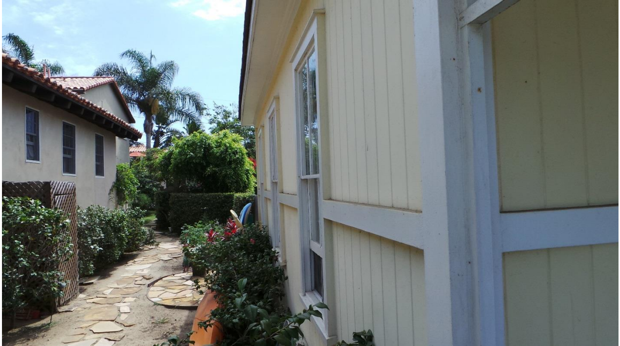
119 10 th Street, Del Mar September 2017 Photograph #49 View south along east façade
