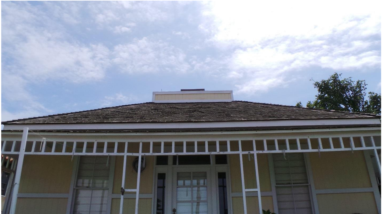
119 10 th Street, Del Mar September 2017 Photograph #5 View of shingle roofing
