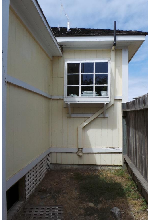
119 10 th Street, Del Mar September 2017 Photograph #47 View north along the east façade
