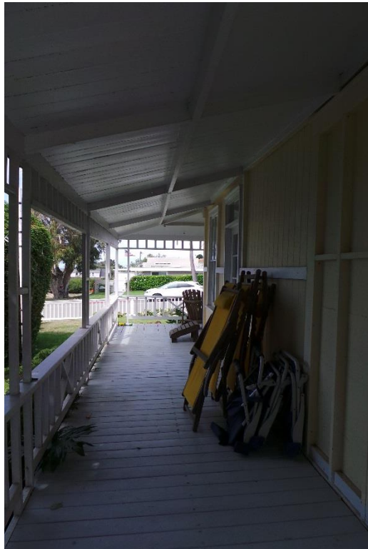
119 10 th Street, Del Mar September 2017 Photograph #22 View north along the west façade
