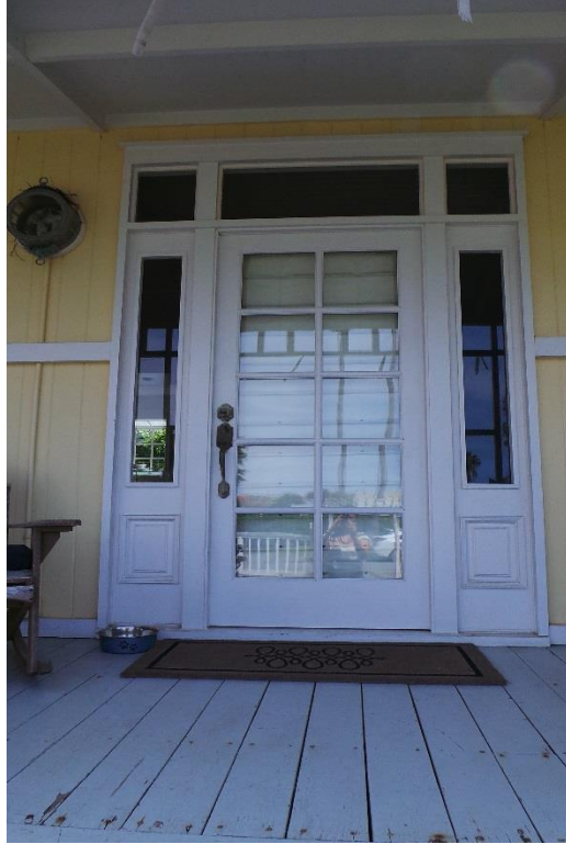
119 10 th Street, Del Mar September 2017 Photograph #11 View of replaced front door entrance
