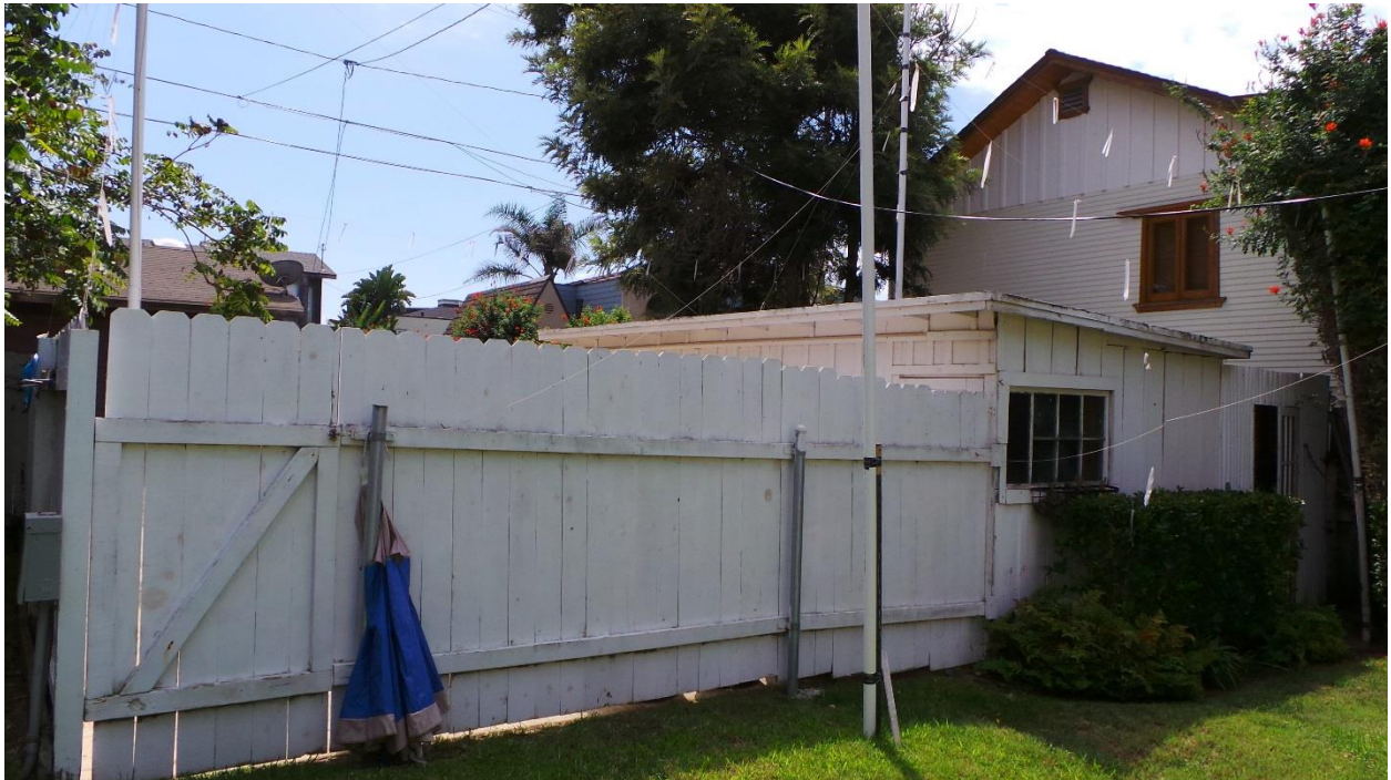
119 10 th Street, Del Mar September 2017 Photograph #50 View of southwest of gate leading to garage in the rear
