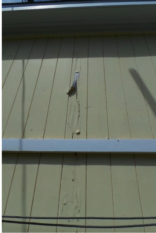
119 10 th Street, Del Mar September 2017 Photograph #43 View of wood surface on rear addition
