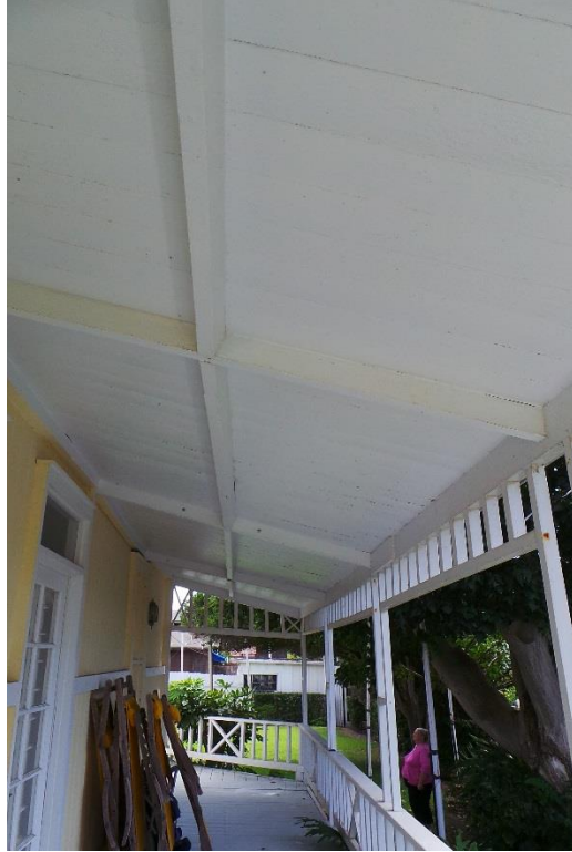
119 10 th Street, Del Mar September 2017 Photograph #19 View of porch roof on the west façade
