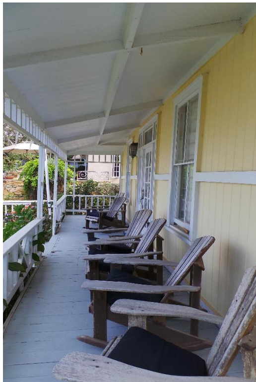
119 10 th Street, Del Mar September 2017 Photograph #16 View east of the north façade porch
