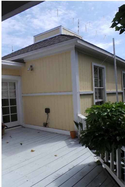
119 10 th Street, Del Mar September 2017 Photograph #36 View southeast of attached rear addition
