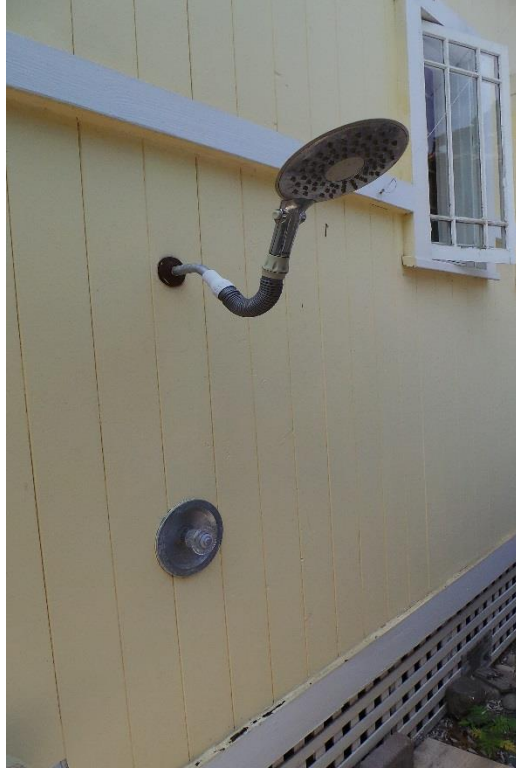
119 10 th Street, Del Mar September 2017 Photograph #45 View of outdoor shower on east side of rear addition
