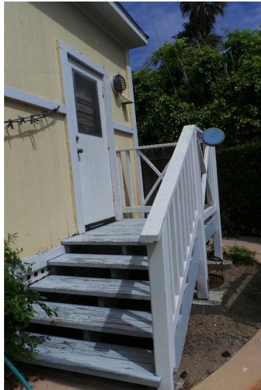
119 10 th Street, Del Mar September 2017 Photograph #42 View of east of staircase leading to rear addition
