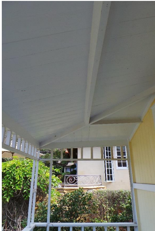
119 10 th Street, Del Mar September 2017 Photograph #14 View east of porch roof
