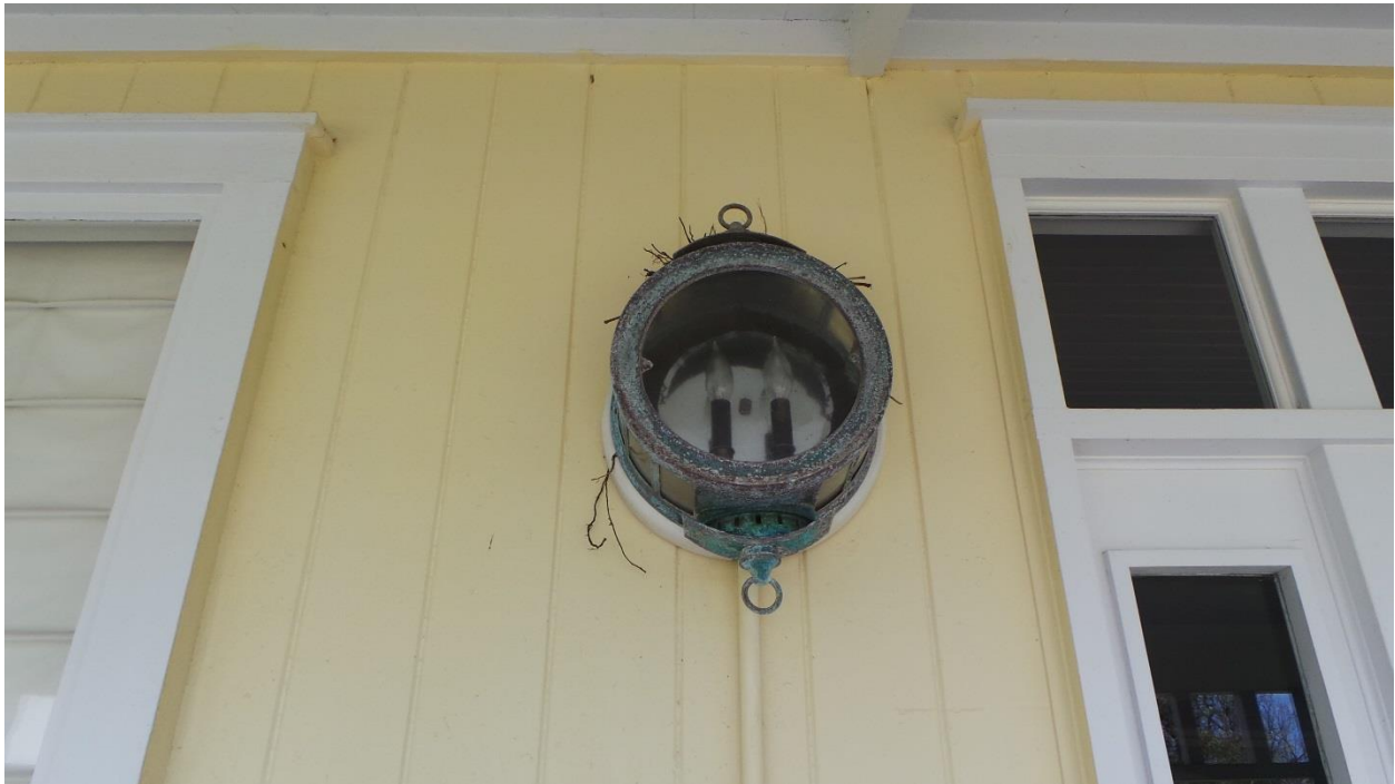
119 10 th Street, Del Mar September 2017 Photograph #10 View of light fixture by main entrance
