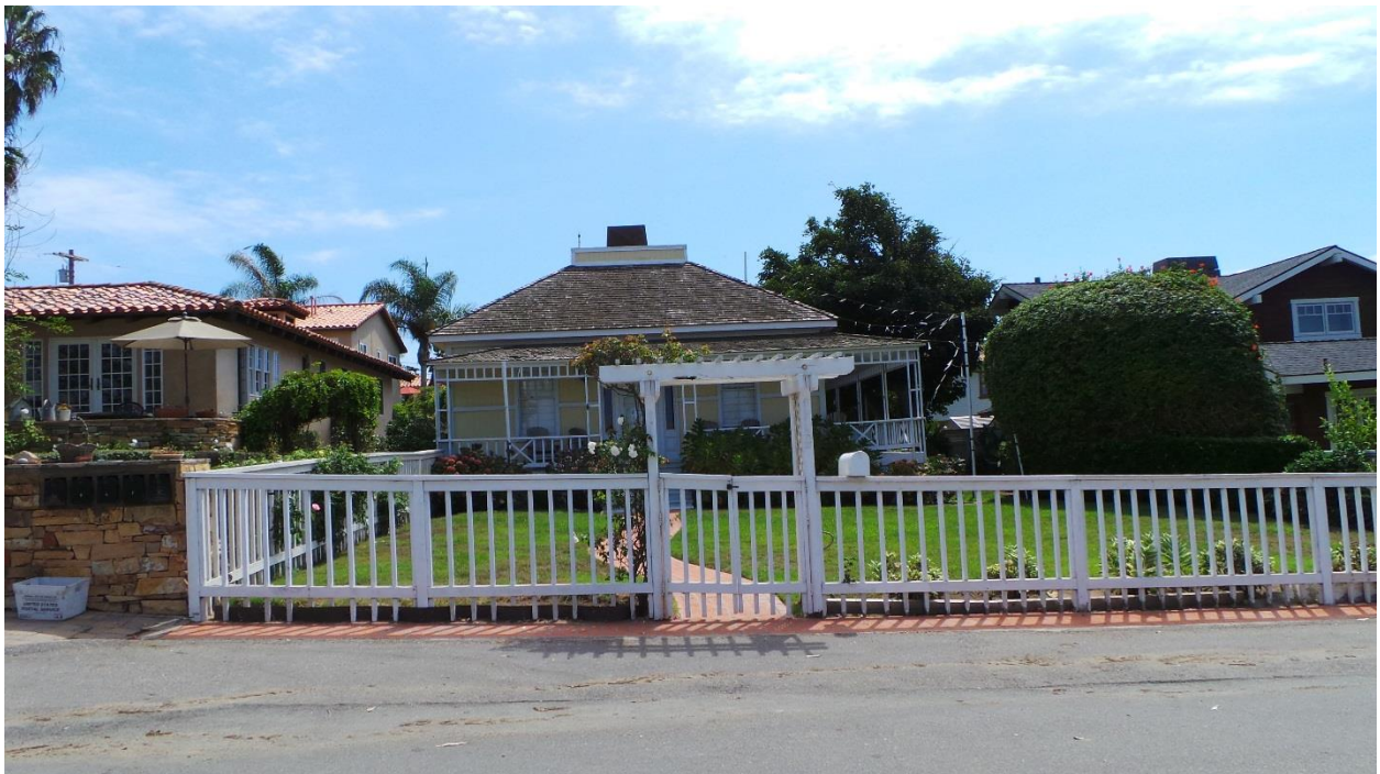
119 10 th Street, Del Mar September 2017 Photograph #2 View South of the north façade
