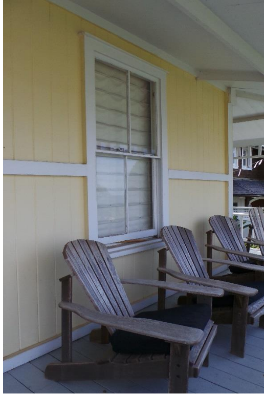
119 10 th Street, Del Mar September 2017 Photograph #17 View of window on the north façade, west end
