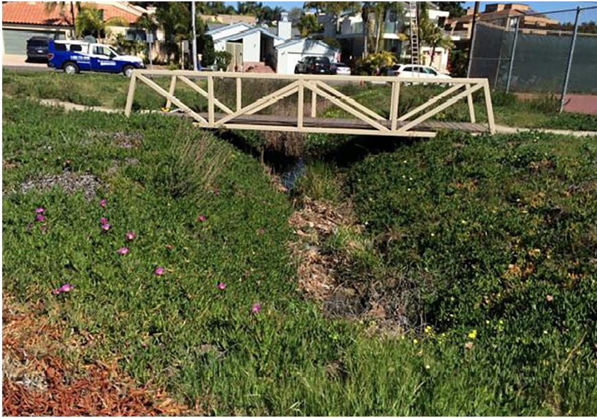
View looking north (downstream) from upstream limits of project site.
