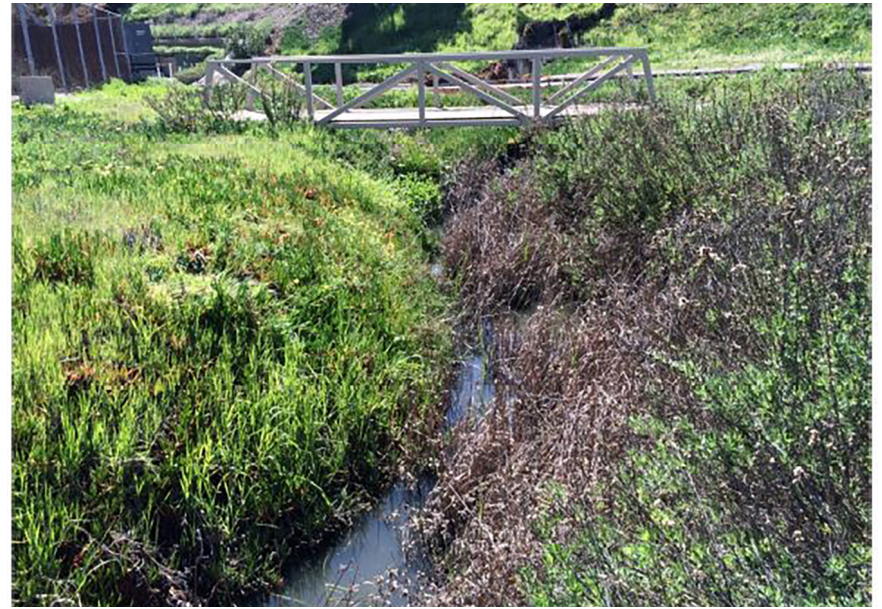
View looking south-southwest (upstream) at the upstream limits of the project site.
