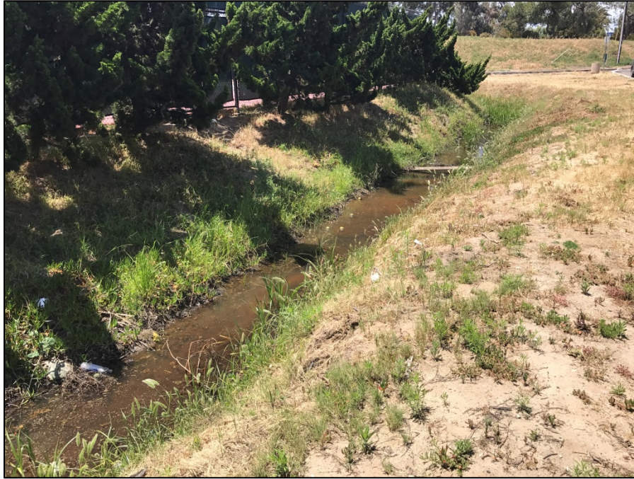
Figure 4 Existing drainage ditch, view west
