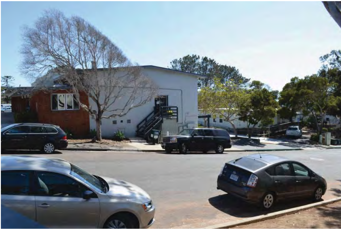
07a_VIEW SOUTHWEST FROM 11TH STREET
