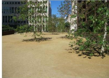
DECOMPOSED GRANITE PAVING W/ STABILIZER
