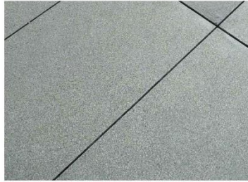
CONCRETE PAVING TYPE 3: INTEGRAL COLOR W/SAND FINISH
