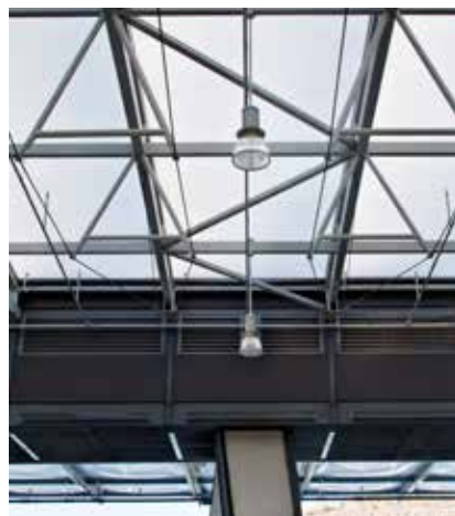
San Ysidro Land Port of Entry: Translucent ETFE pillows reduce the need for daylight.
