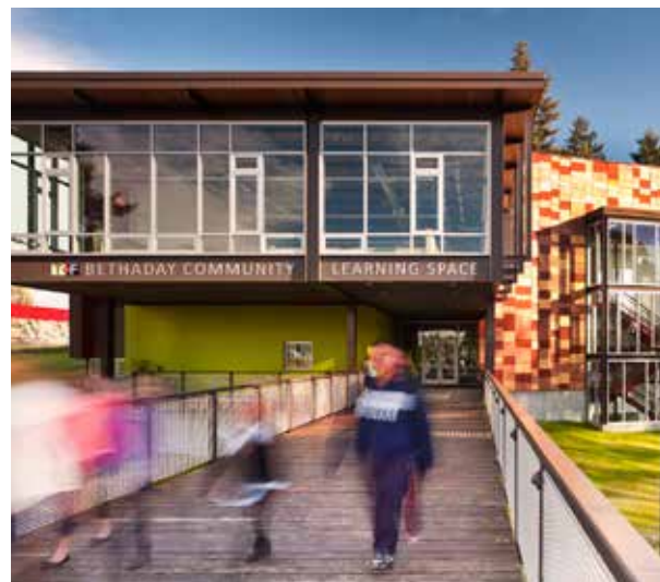
Technology Access Foundation
