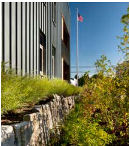
Fire Station 39: Stormwater infiltration with recycled granite curbstones
