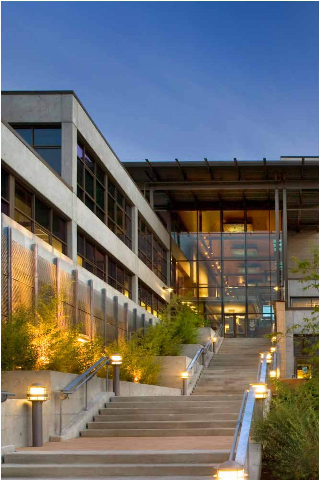
Main entry at the Kitsap County Administration Building
