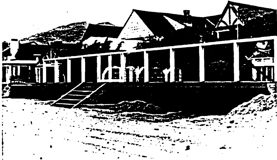
A. TIMBER PILES WITH TIMBER LAGGING, MALIBU
