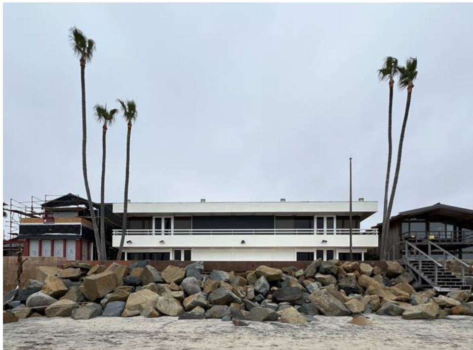
EXHIBIT 2.1-1: 2936 Camino Del Mar (looking east from beach)
