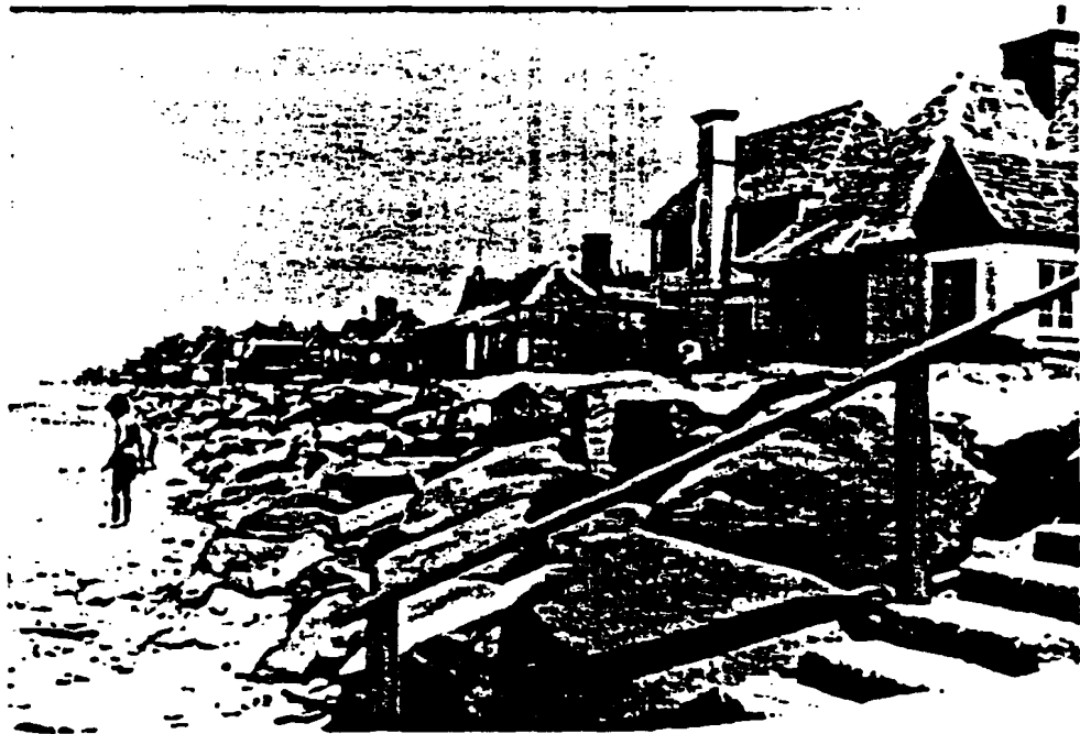
B. STONE REVETMENT, SAN MALO BEACH AT OCEANSIDE
