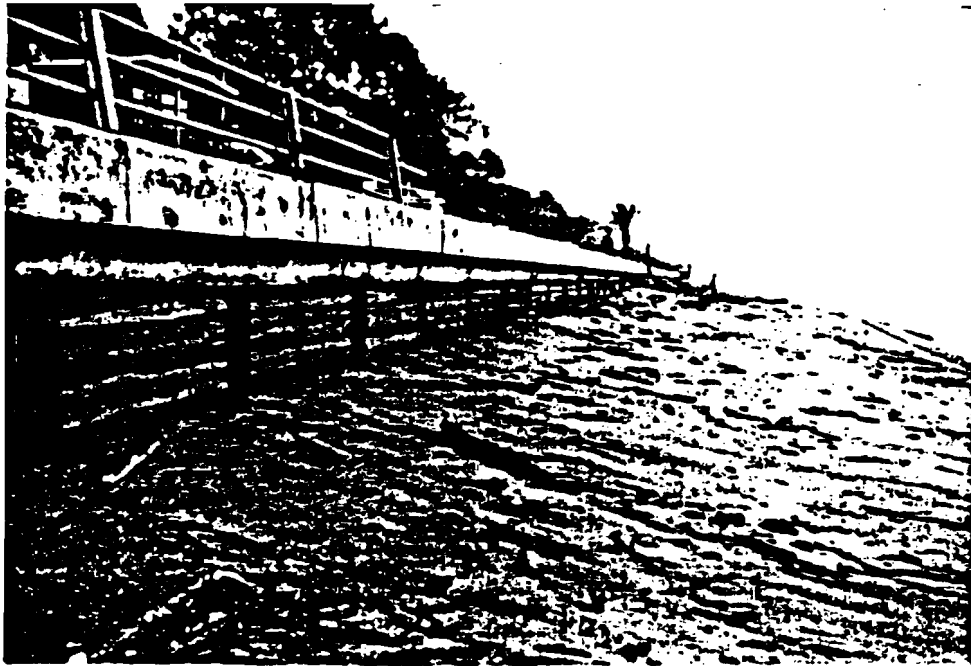
B. STEEL H-PILES WITH TIMBER LAGGING AND CURVED CONCRETE CAP, RIO DEL MAR, SANTA CRUZ COUNTY
