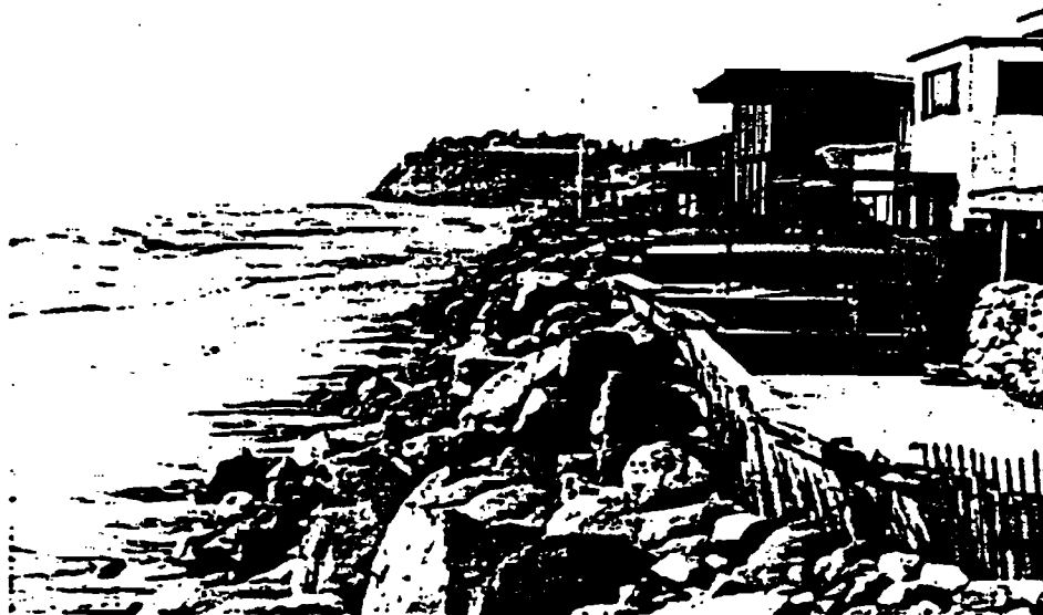
A. 26th STREET LOOKING NORTH
