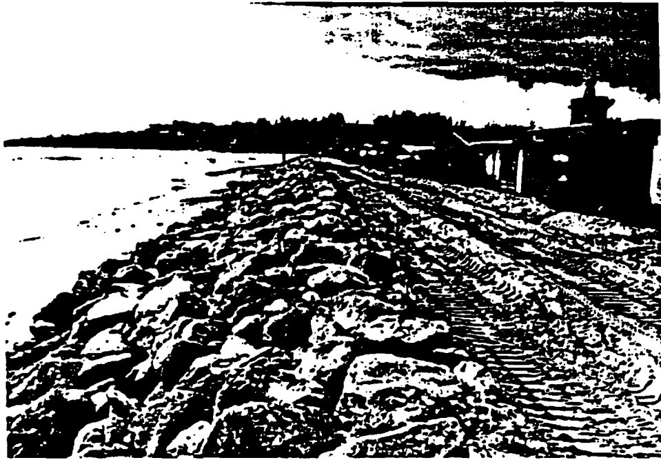
A. STONE REVETMENT, SEADRIFT AT STINSON BEACH
