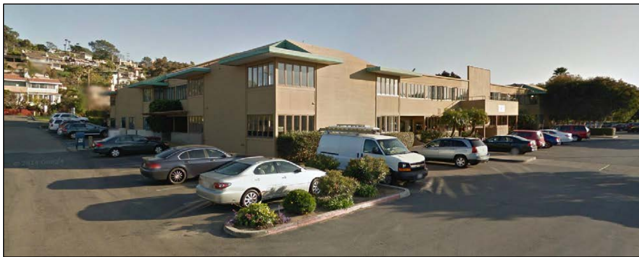
View of Southfair, from the westerly parking lot looking east-southeast.
