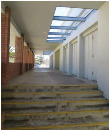
GRAY ROOM 3,020 GSF of unusable space
