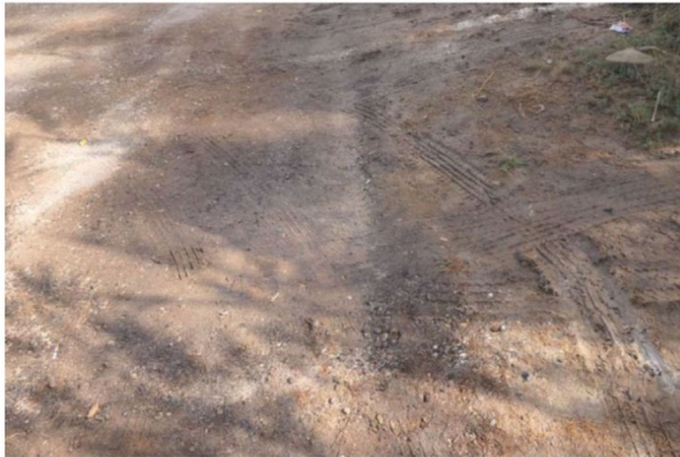
Photo 2. Close-up view of muddy and moist soil in the area shown in Photo 1, taken on 11-7-17.
