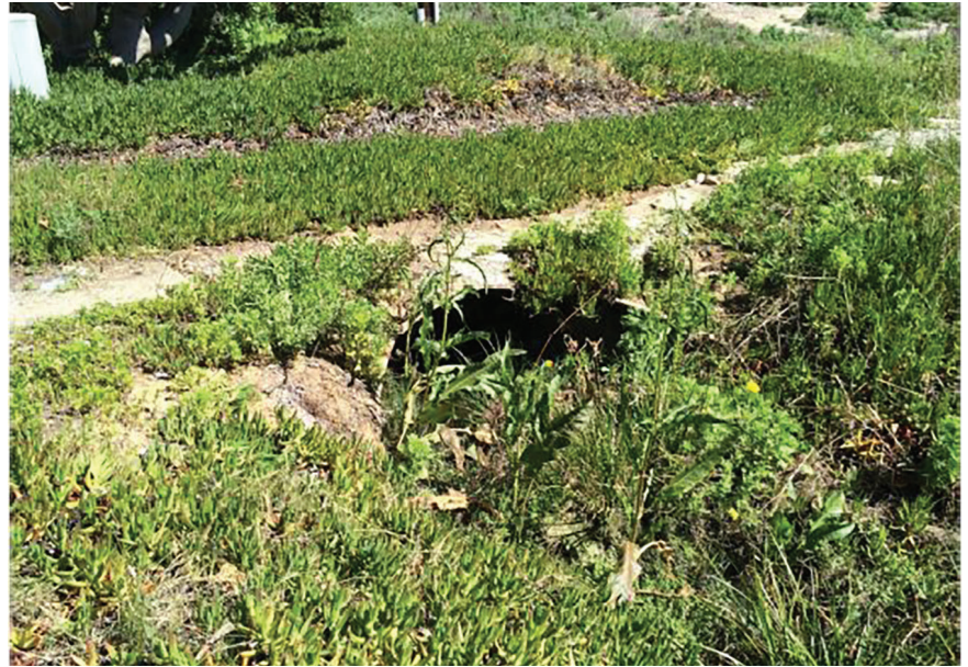
View looking northwest (downstream) at the culvert outlet.
