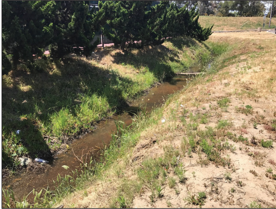
Figure 4 Existing drainage ditch, view west
