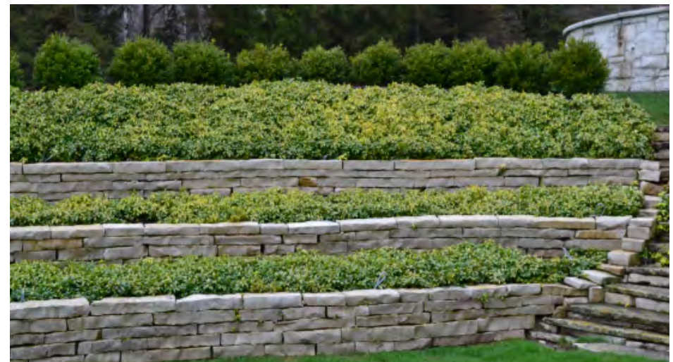
Planting pockets integrated into the terraced retaining walls.
