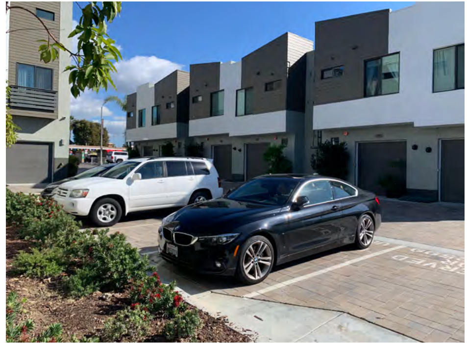
Uncovered parking at the rear of the parcel with landscaped screening.
