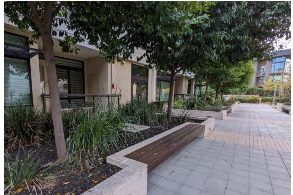
Public walkway paved with permeable pavers.
