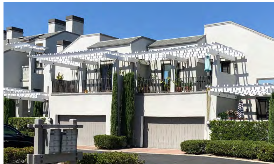
Recess garage doors to add shadow.
