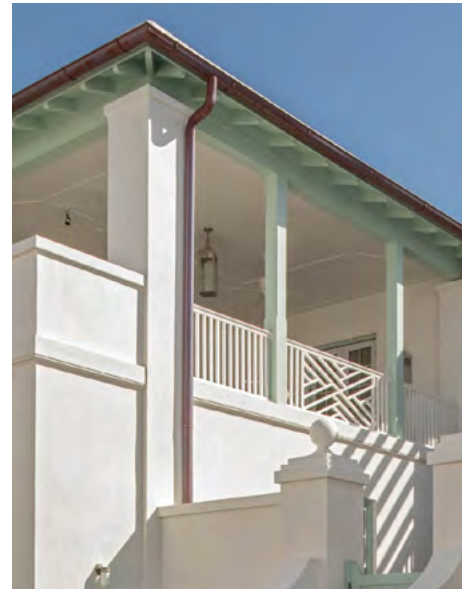
Decorative gutters matching roof.
