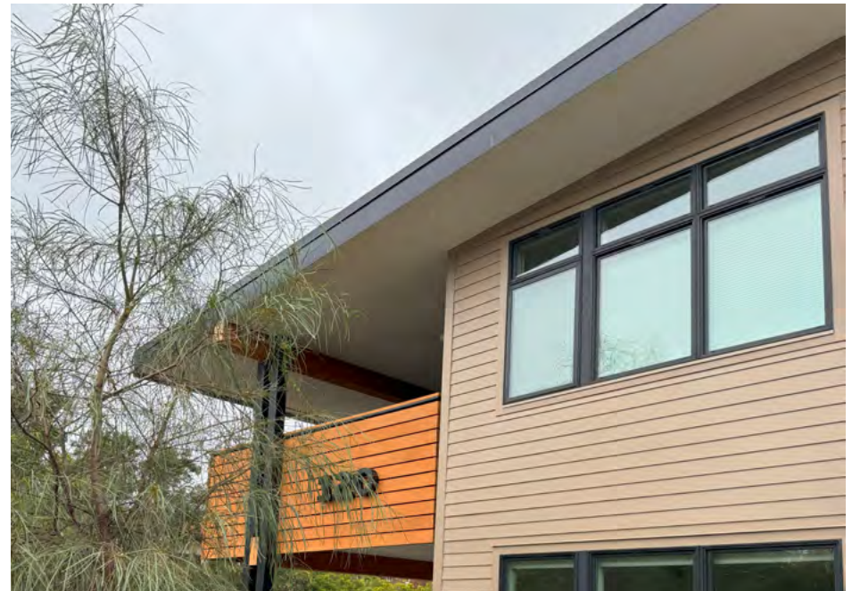
An example of a roof overhang.
