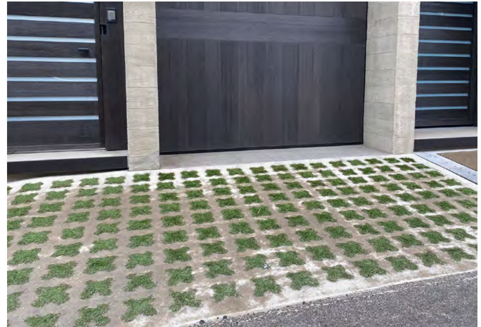
Permeable paving at a parking garage entrance.
