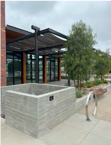
Screening of utilities with solid walls.
