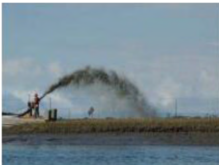
Figure 6.1 Sediment Placement on the Marsh at Seal Beach
