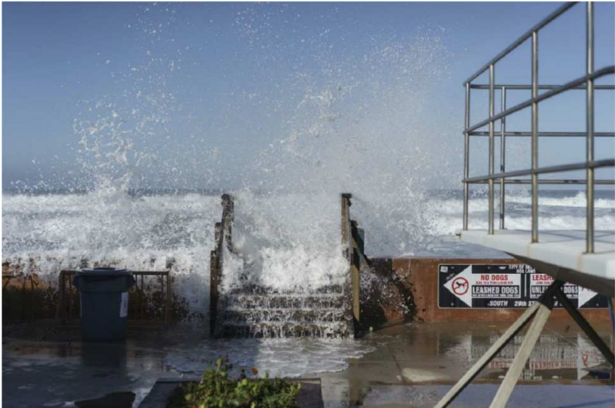
Figure 9.1 Overtopping in Del Mar on March 8, 2016
